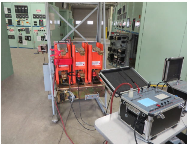
Figure 3: VI Vacuum Test (MAC Test)
